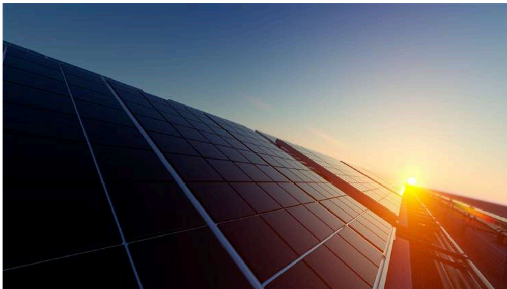
A solar farm
